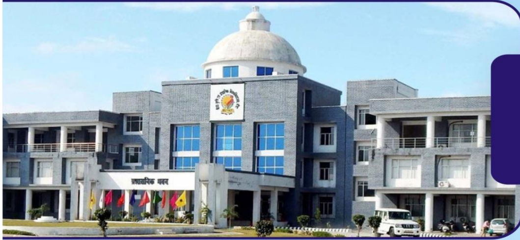
Administrative Building BUA&T, Banda
